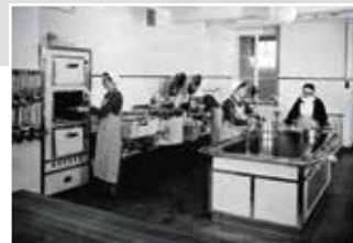
Cooking installation in Kloster 1960
