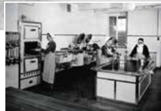
Cooking installation in Kloster 1960
