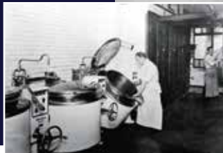
First generation of tilting boiling pans 1934
