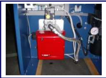
When there is a **modulating burner (BS3/M)** installed, the **lowest possible power output must be regulated below 60kW !!!**
