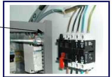
When the connection cable is connected, the main switch can be moved to position "1" and the direction of movement of the motors must be checked (to prevent damage).
